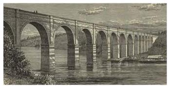
is a National Historic Landmark, and a National Historic Civil Engineering Landmark. High Bridge was originally built with fifteen arches. In the 1920s High Bridge was reconstructed, replacing the central spans with a single steel span.
