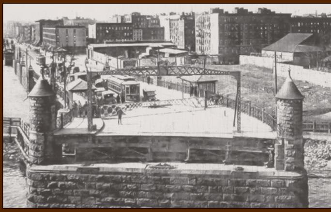
With the swing span open, an electric trolley is stopped on the Manhattan approach, as viewed from the open swing span of the former Willis Avenue Bridge – ca.1930.
