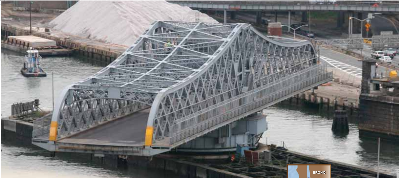
Former Willis Avenue Bridge with swing span opening for navigation.
